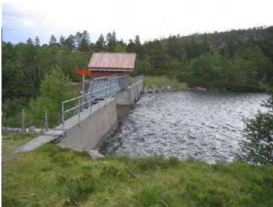
Dam Riksheimdalen (Foto: SE)
